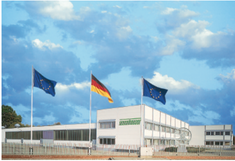
Production plant in Neuenhaus
